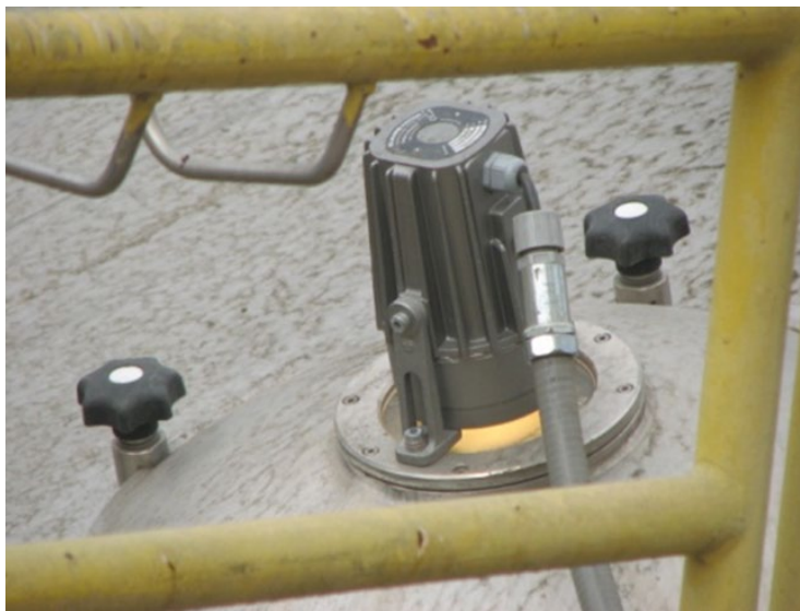
Figure 2. High intensity discharge lamp lights the inside of the whirlpool tank.
